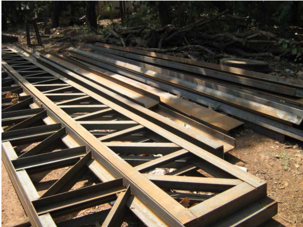
Truss work for workshop building
