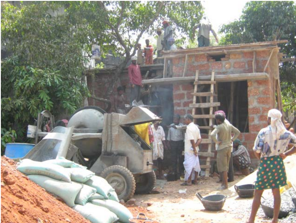
Construction of office building
