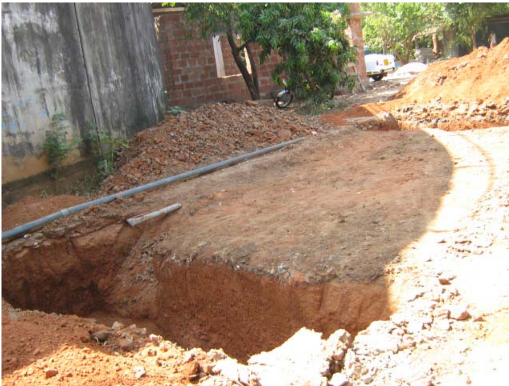
Weigh bridge – earth work excavation completed
